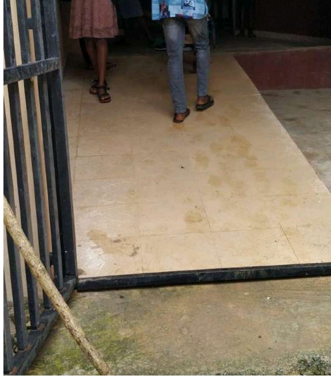
Plate 16: The ramp from the medical records room to the external walkway
