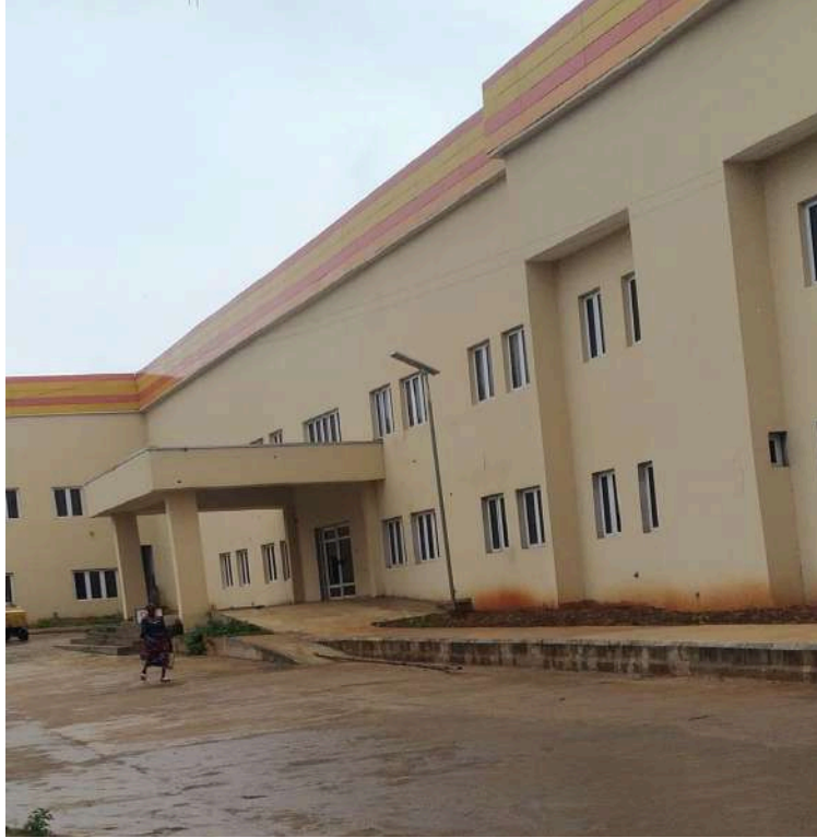
Plate 1: The new building's entrance with ramps
